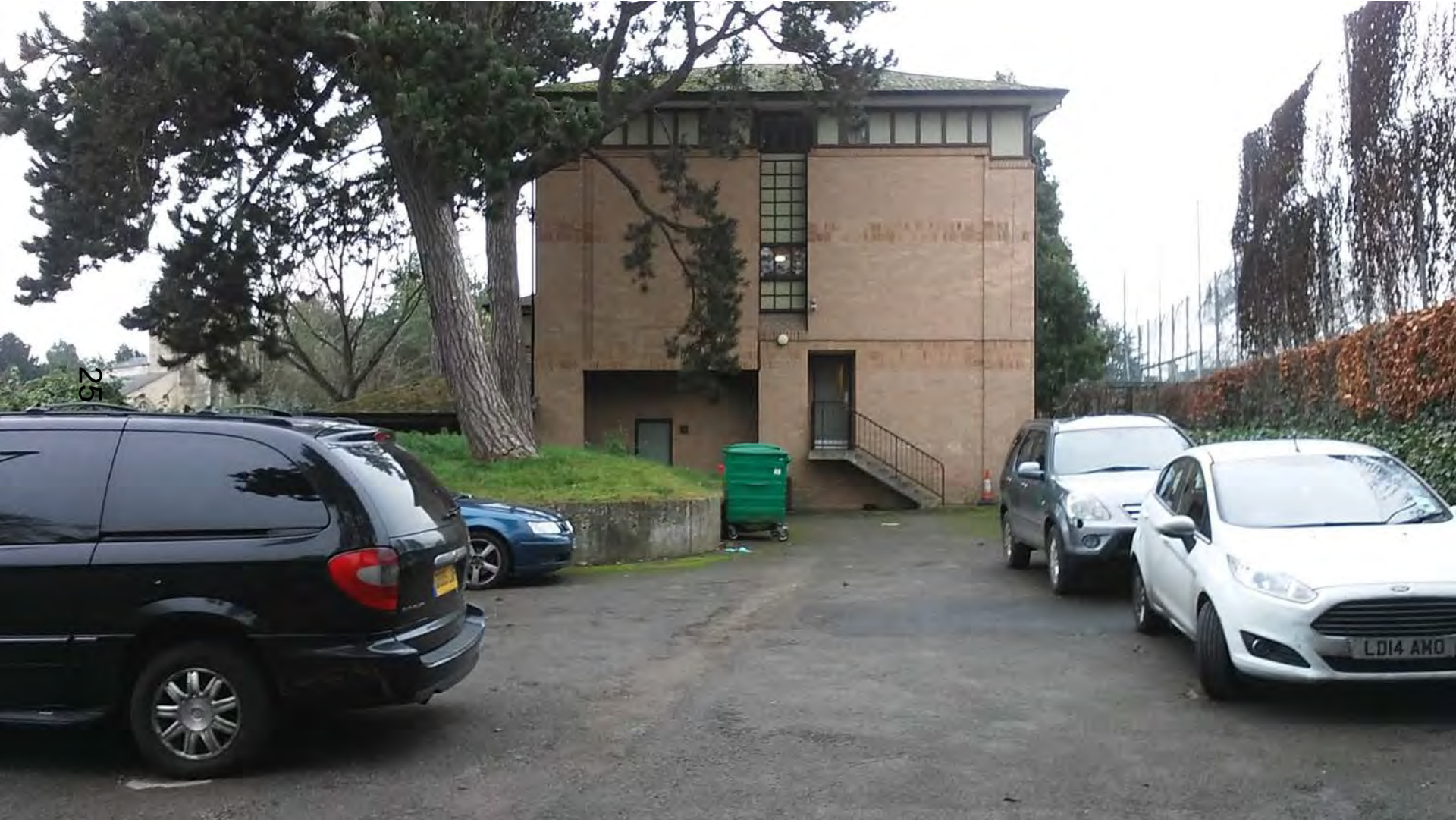
Existing car parking area adjacent to the Dellal building
