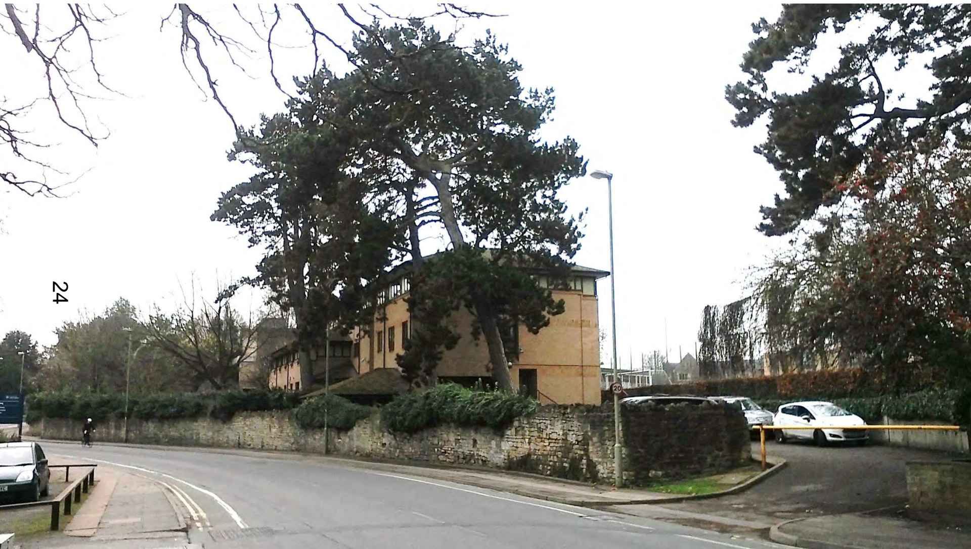
View from north towards the Dellal Building showing pines trees
